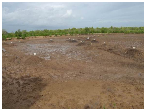
Figure 13. Pond excavations as of Feb 2010
