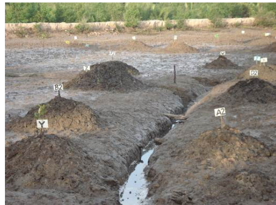
Figure 4. Excavated channel, following original stream to improve hydrology, with labelled hills for mangrove growth and monitoring
