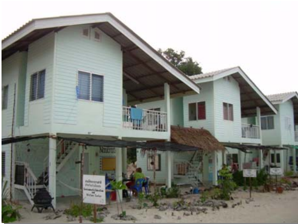
The walkway connecting two houses was finished. (February 2009)
