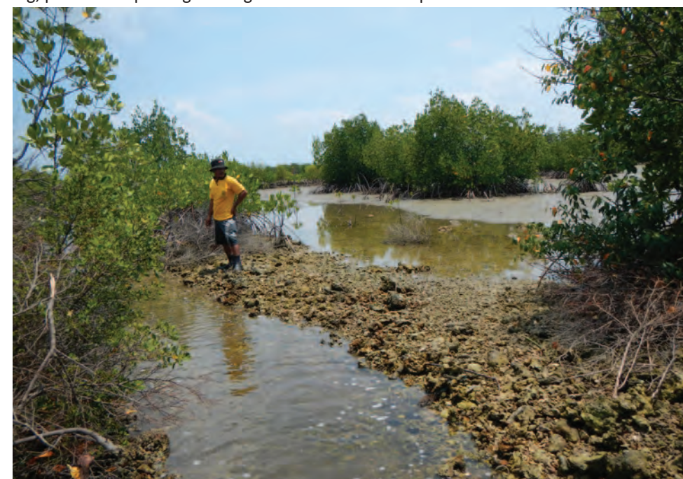
Fig 5.18 Hydrological Disturbance - Although this dike wall was levelled during initial rehabilitation, it is still high enough to block drainage of the pond (background) into the tidal creek (foreground). After identifying continued hydrological disturbance during monitoring, plans for improving drainage need to be made as part of mid-course corrections.
