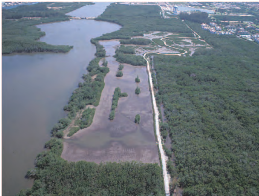
Fig 8.15 The intentional design of open water refugia in a mangrove rehabilitation project, increases fisheries habitat and can speed up the achievement of a functional fisheries equivalent, and wading seabird feeding habitat, common objectives of mangrove restoration projects.
