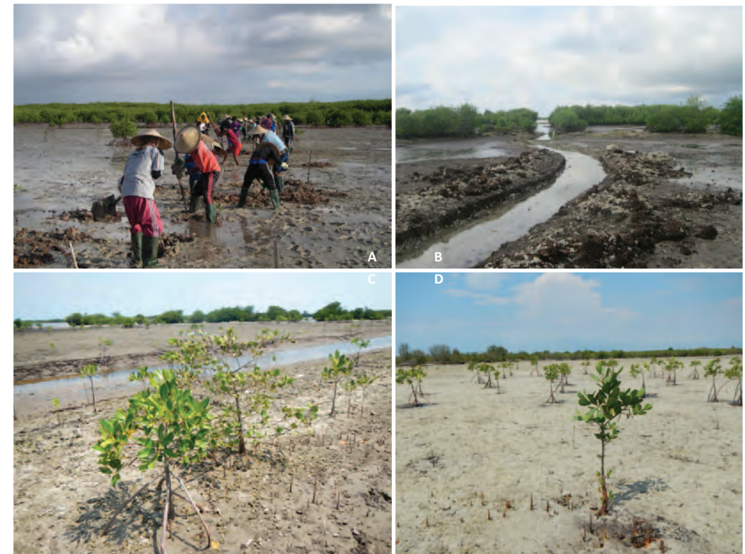
Fig 10.12 A) Members of the Womangrove group hand-dig a 1.2 km tidal channel, to facilitate drainage of disused shrimp ponds at Lantang Peo village as part of mid-course corrections 12 months after initial rehabilitation (above left). B) The resultant, meandering tidal channel. Material on the side of the channel was eventually moved away into island-like mounds in the middle of ponds (above right). C) Natural recruitment of Sonneratia alba and Rhizophora apiculata 32 months after initial rehabilitation (bottom left). D) The middles of some ponds are being recruited as well, again by Sonneratia alba and Rhizophora apiculata (bottom left).
